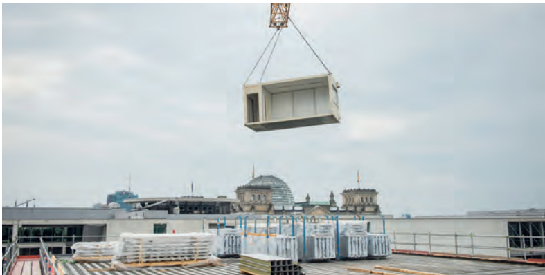
Luisenblock West building site: a module is lifted onto the site by crane.
